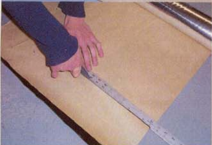
5. We then transferred those measurements to the Brown Bread and carefully cut the material with a razor knife using a yardstick as a guide.
