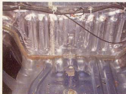
12. After applying the mat (which once again required no heat) we marked the location of the holes, pressed them out and re-installed the wiring harness. Notice the holes that had been drilled in the spare tire well. Rather than apply more mat and add unnecessary weight, we filled them with silicone to keep water from getting in and damaging anything.
